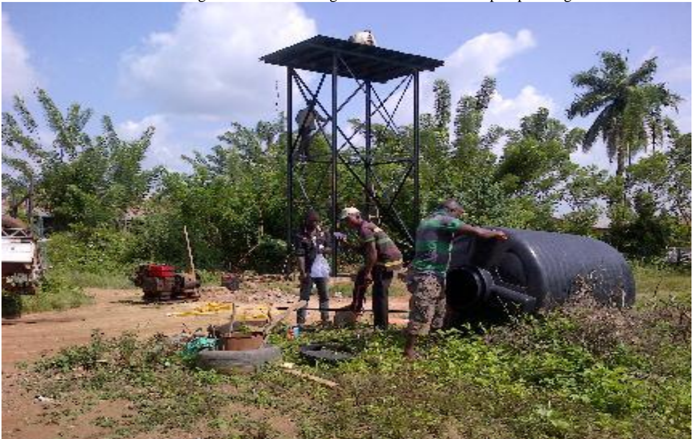
Overhead Stanchion construction process
